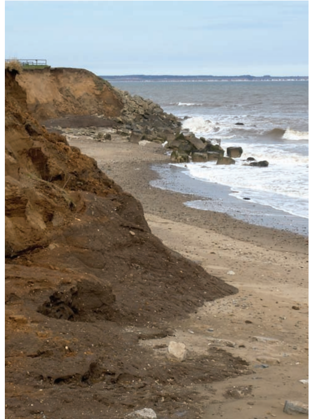
Coastal erosion at Barmston, East Riding of Yorkshire
