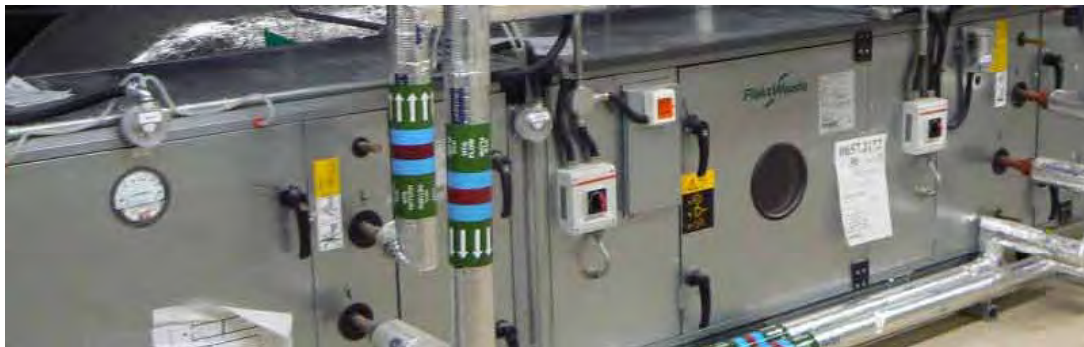
Combined Heat and Power
