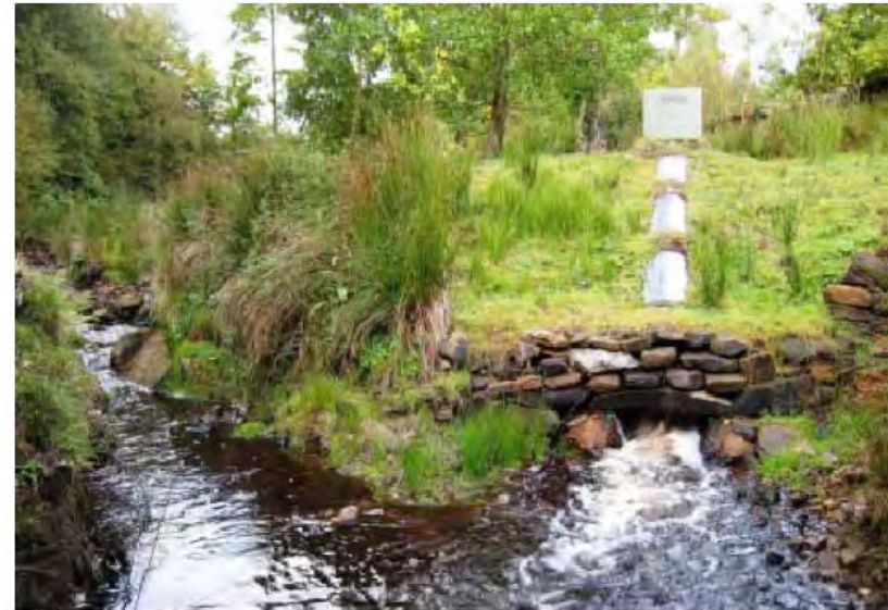
Figure 24 Bonfield Ghyll hydro facility in the North York Moors National Park (Source: Case study, Mann Power Consulting Ltd)
