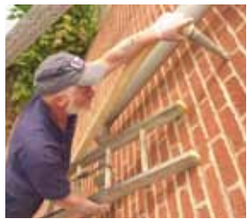
insulating the walls
