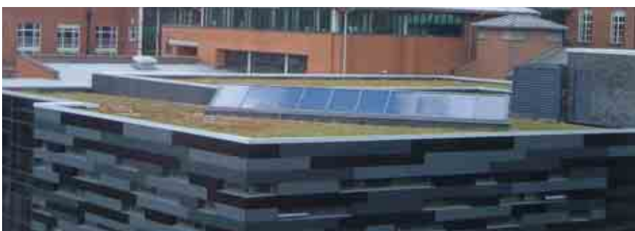
Green roof, Performing Arts Building, Leeds. Designed by Ian Tod and Company
