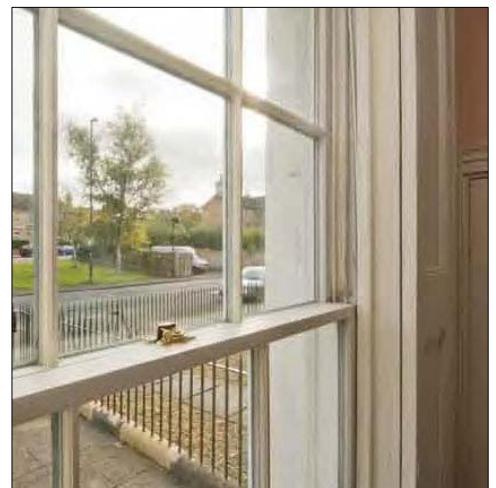
Timber slim-profile double glazing is hard to spot. It is ideal for most traditional homes in Bath
