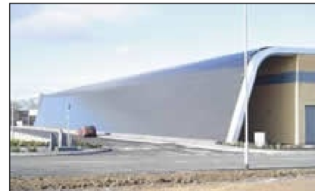
Standing seam roof
