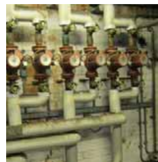
Duty and standby circulation pumps serving different zones.
