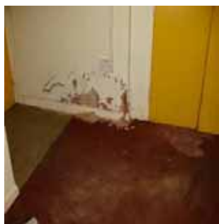
Water ingress at basement level.
