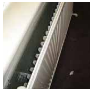
Reflective foil behind panel radiator.
