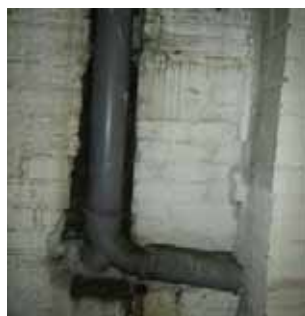
Drainage pipework recessed into wall.
