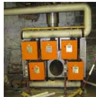
Modular gas fired boiler.
