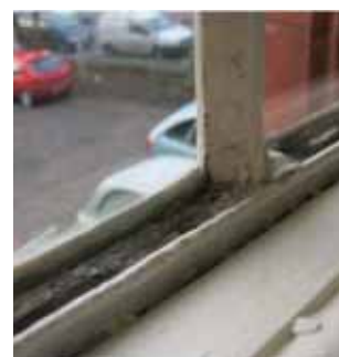
Typical poorly maintained window frame to offices
