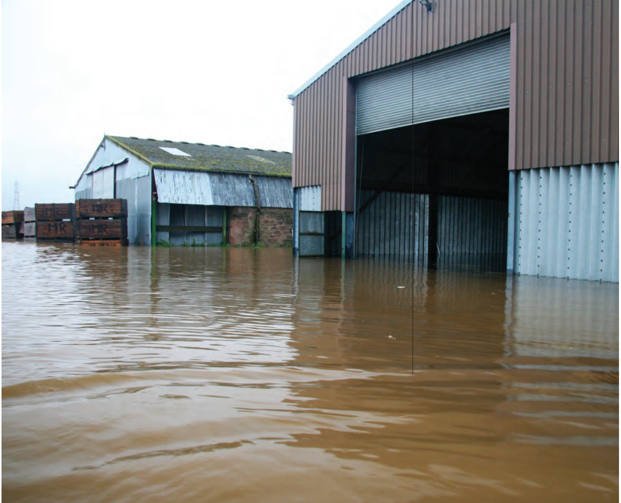
Intense rainfall led to the flooding of Fenton farm
