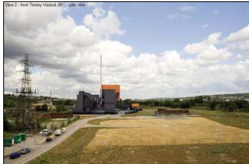
View 2 - from Tinsley Viaduct (M1) - side view
